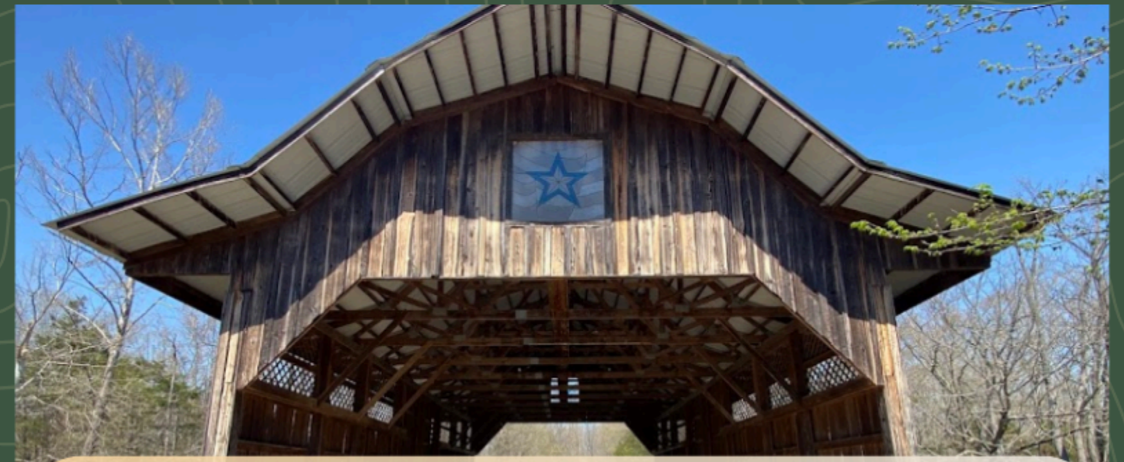
Hackney Creek Covered Bridge
