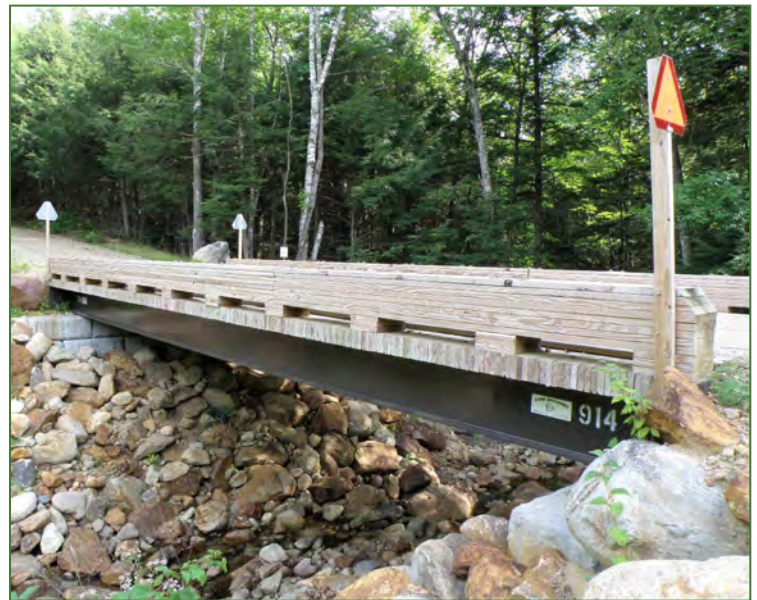
Nearly all bridges are new construction.
